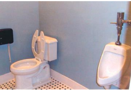
The mens restroom after the renovation.
